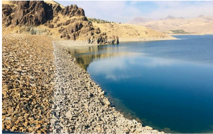
Fig. 1. Gheshlagh Dam (Vahdat) in Sanandaj City.
